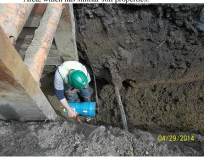
C900 pipe being installed during Phase 1
